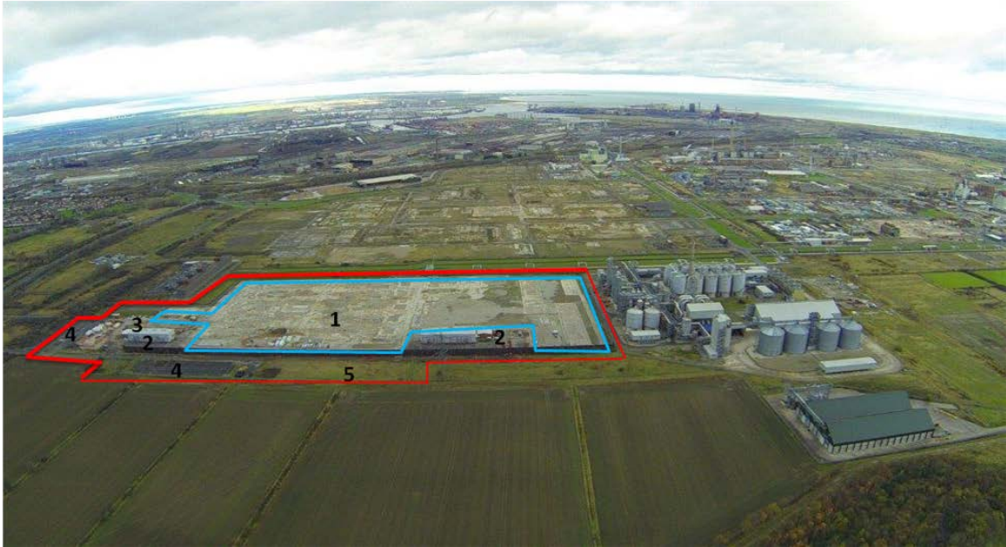
Figure 1. The application site in its wider context
